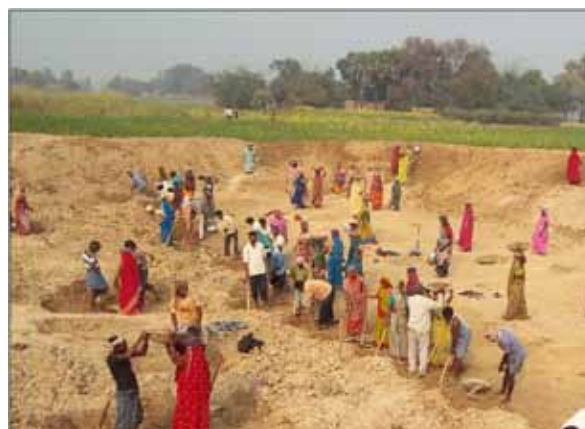
Work at a PANI operating village
