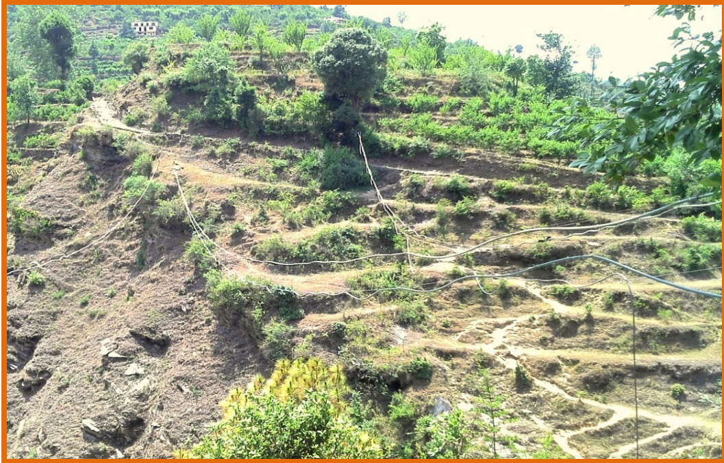
Image: 6.3 Swinging Pipelines carrying irrigation water from gadhera
