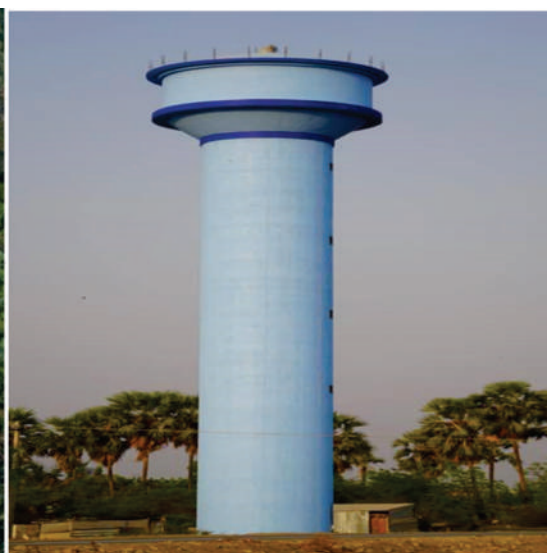
200 KL OHBR at Seetharampur Palair segment
