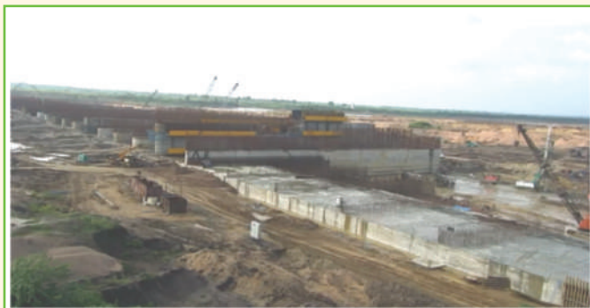
Annaram Barrage under construction
