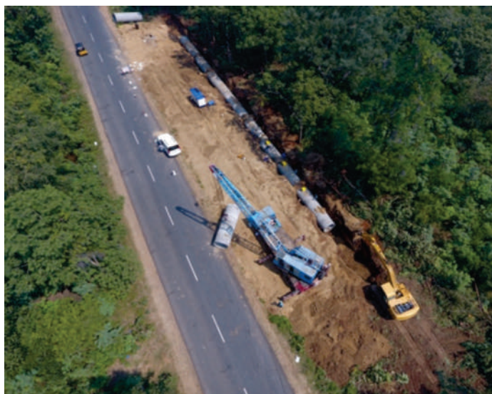
1500-mm-diameter PCCP pipeline Godavari Dummu-gudem segment
