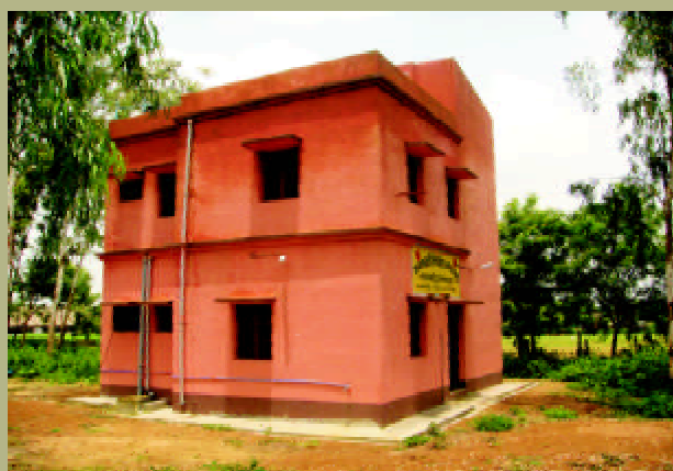
Kankabati Gram-Panchayat Headquarters Sub-centre in Medinipur Sadar Block
