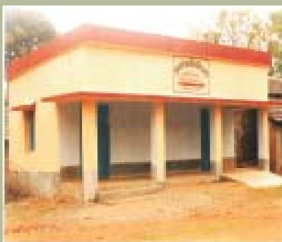
Primary School building at Nayagram
