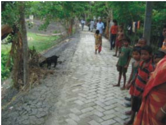
A Brick flat soling road constructed under NREGS
