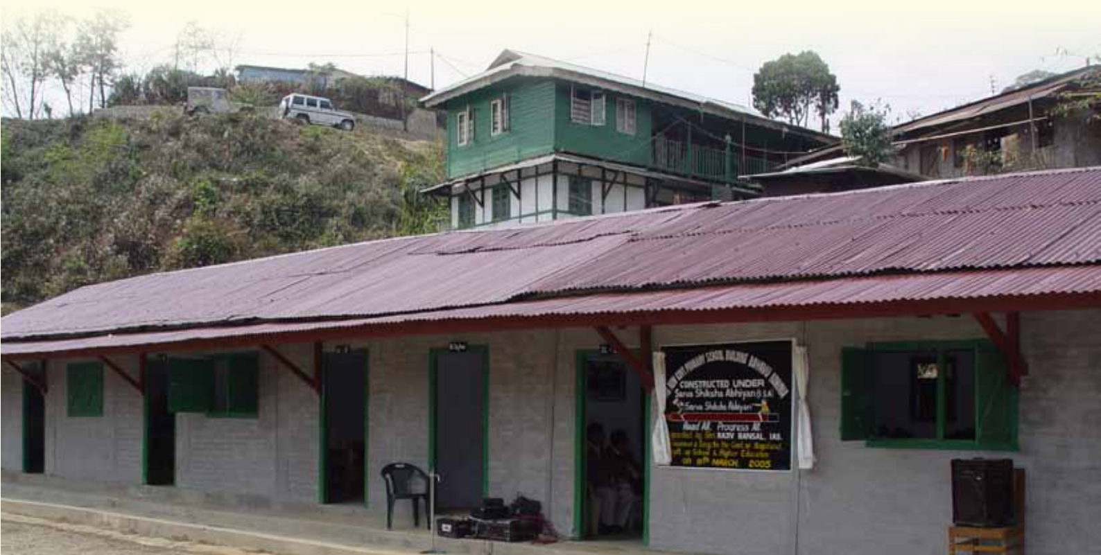
A school constructed under SSA Scheme at Bayavü
