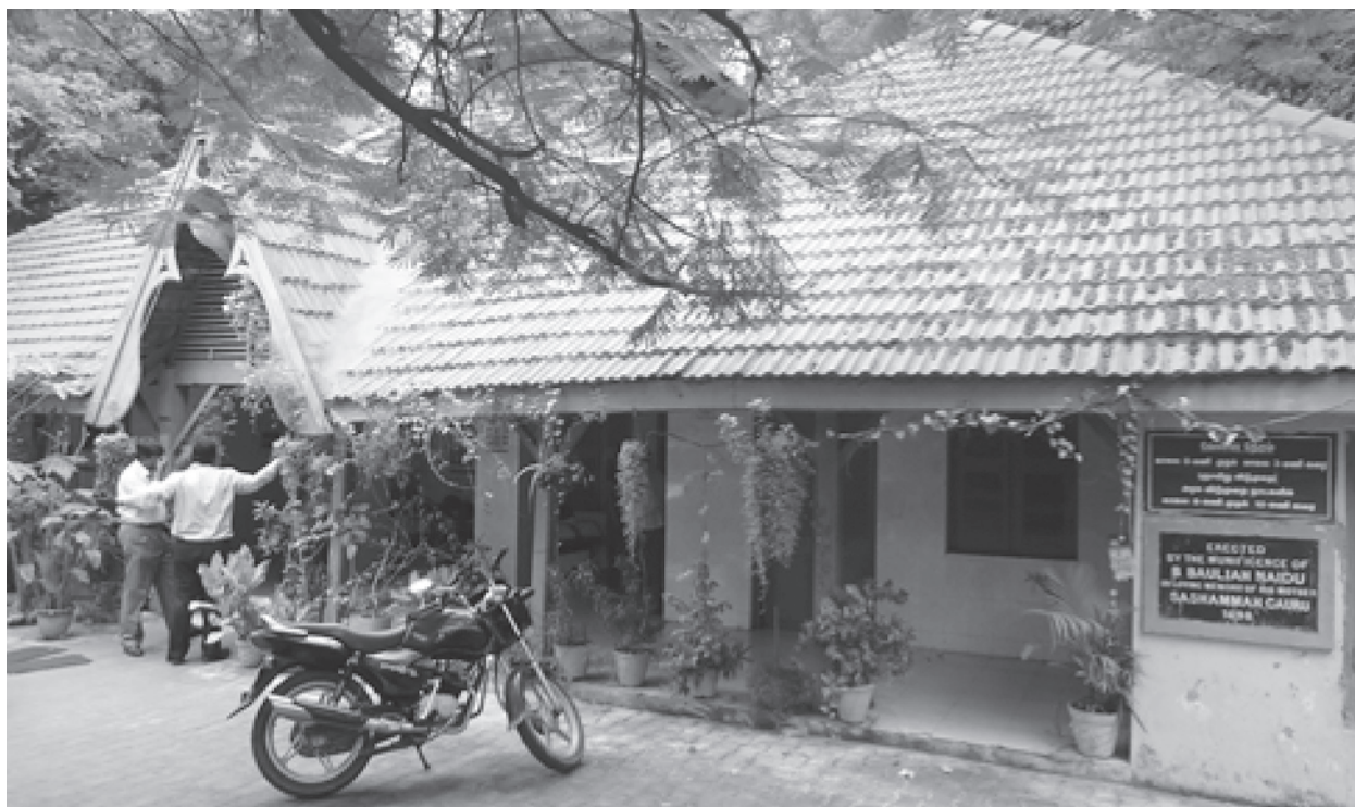
Figure 1. Shri Baliah Memorial Urban Primary Health Centre for Senior Citizens, Rottler Street, Chennai. Photo Credit: Prathibha Ganesan.
