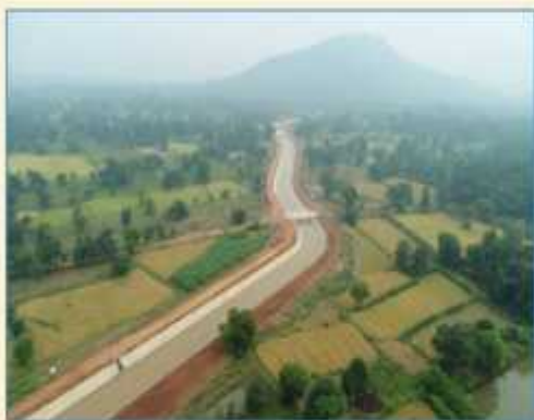
Upper Indravati Lift canal
