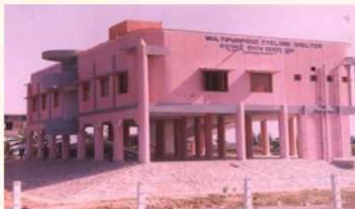
Multipurpose Cyclone Shelter Source: OSDMA
