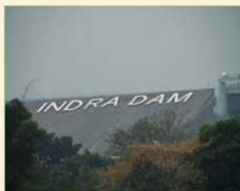
Lower Indra Irrigation Project
