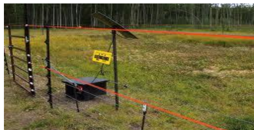
Solar Powered Battery Fencing
