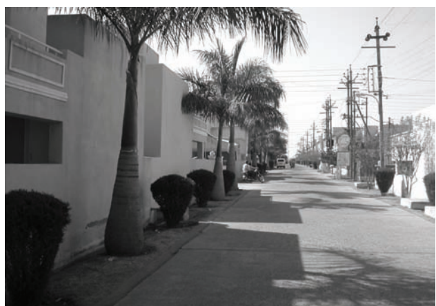
Concrete gives new life to internal roads
