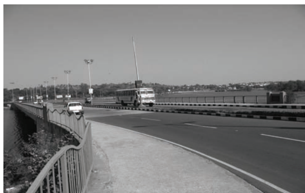
City roads after renovation bring comfort to commuters
