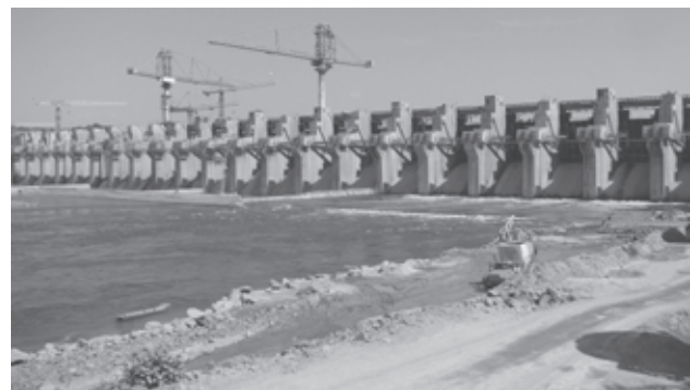
Construction of dam in progress
