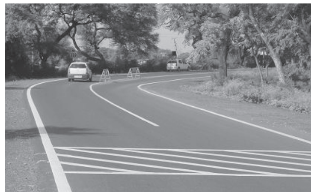
Improvement in road quality— State Highway constructed by MPRDC
