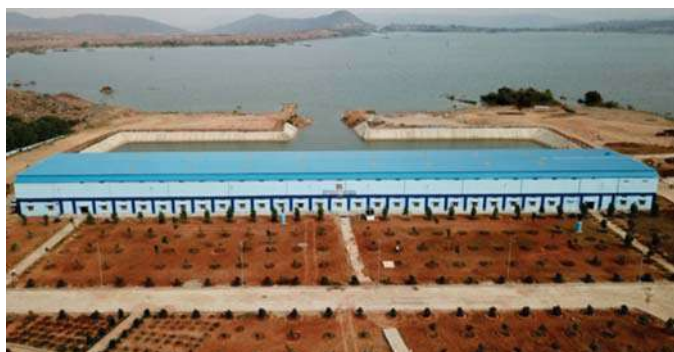
130.25 x 36m Intake Well at Yellore – Yellore Segment
