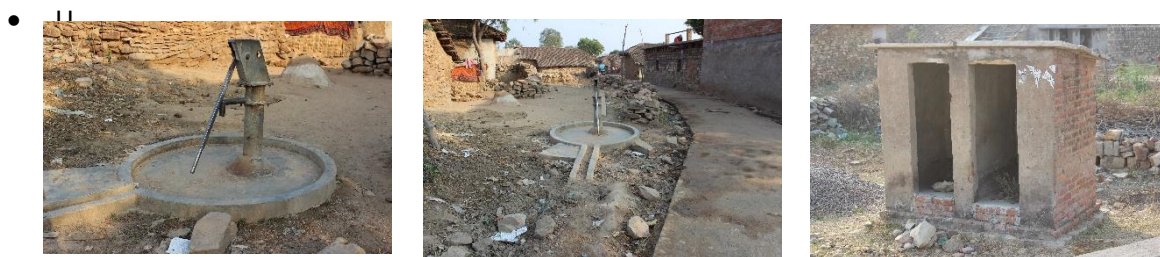
Dysfunctional hand pumps due to steep drop in ground water level, and dysfunctional abandoned toilet Location: Chheria Khhur/Buzurg
