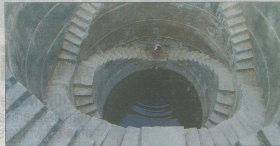
■ This ancient step-well famous as Supa Ki Bawri was built by Chandelas. It has 178 steps in three concentric circles leading up to the water. While most of the similar bawris are dilapidated and retain their original lime plaster, this one has been renovated with cement plaster. PANKAJ JAISWAL/HTPHOTO
