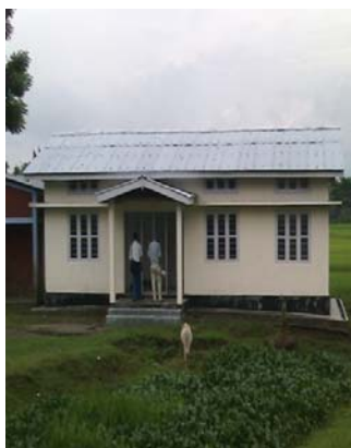
Newly constructed Khanajan Sub Centre in Assam
