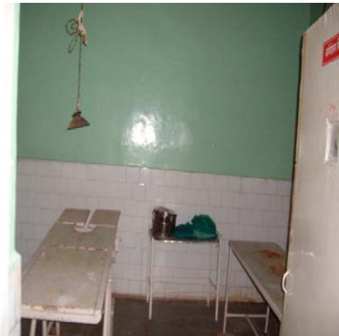
Operation Theatre at PHC-Kendur, Distt. Pune, Maharashtra
