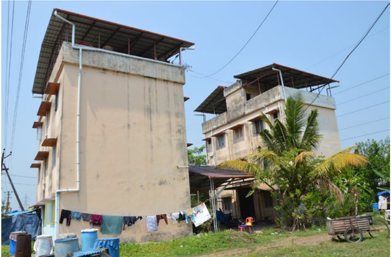
Two apartment blocks were built to house a third of the IDPs displaced by the Perandur Canal in Kochi, Kerala. The apartments are on the outskirts of Kochi and residents now face a long and expensive commute to jobs. See case study on page 29. Credit: IDMC, March 2016
