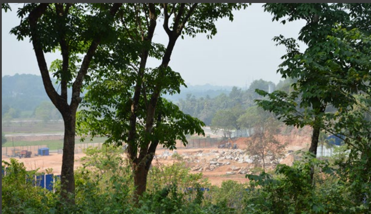
Resettled families displaced by the Smart City in Kochi, Kerala now look over a construction site on their former land. Local resettlement has enabled residents to maintain community ties and maintain proximity to schools and healthcare facilities, however the loss of jobs dependent on agricultural land have not been compensated. See case study on page 30. Credit: IDMC, March 2016
