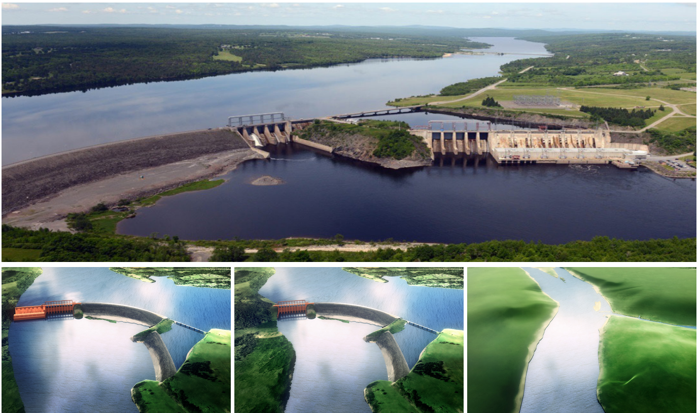
Figure 11: The Mactaquac Hydroelectric Generating Station Dam (actual current view- top) and the options considered for its renewal/removal: Repowering (construction of the new powerhouse and other components – bottom left); Maintaining the dam as a water control structure without power generation – bottom middle, and Removing the dam to ensure a free-flowing river - bottom right Credit and Source: New Brunswick Power 2013; https://www.nbpower.com/en/about-us/projects/mactaquac-project/resources/
