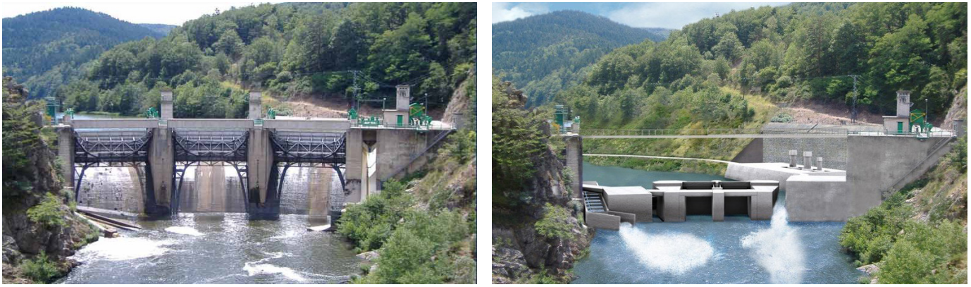
Figure 10. The Poutès dam before (2015) and after partial removal in 2021 (photomontage). Photo credit © EDF Hydro
