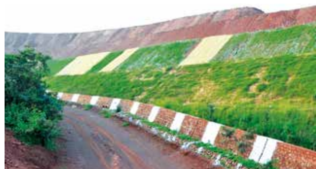
Geo matting of Over Burden of Iron Ore Mine in Karnataka
