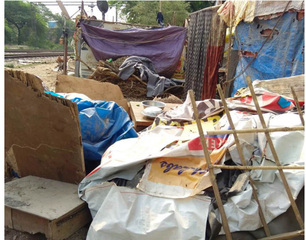
Site of demolition, Shakur Basti, Delhi
