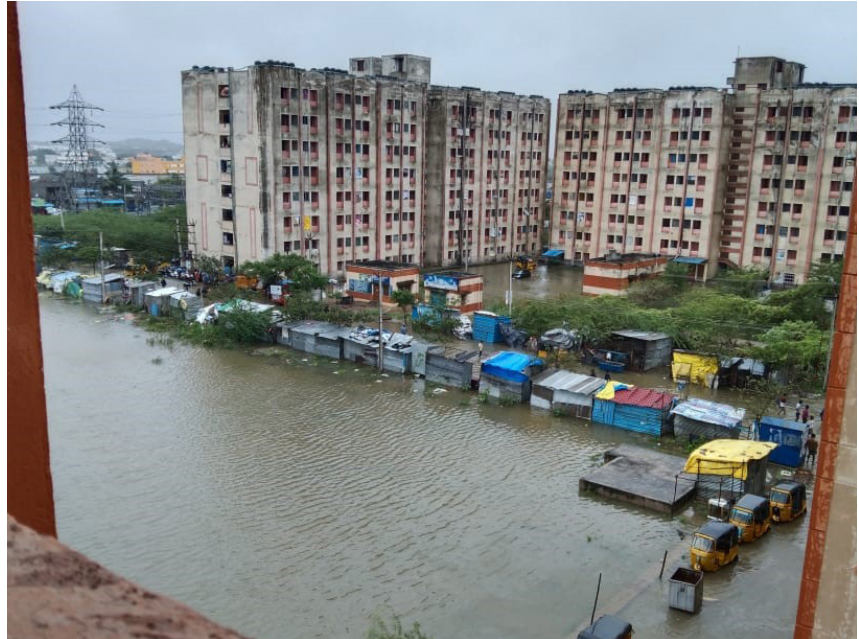
Flooded resettlement site of Perumbakkam, Chennai
