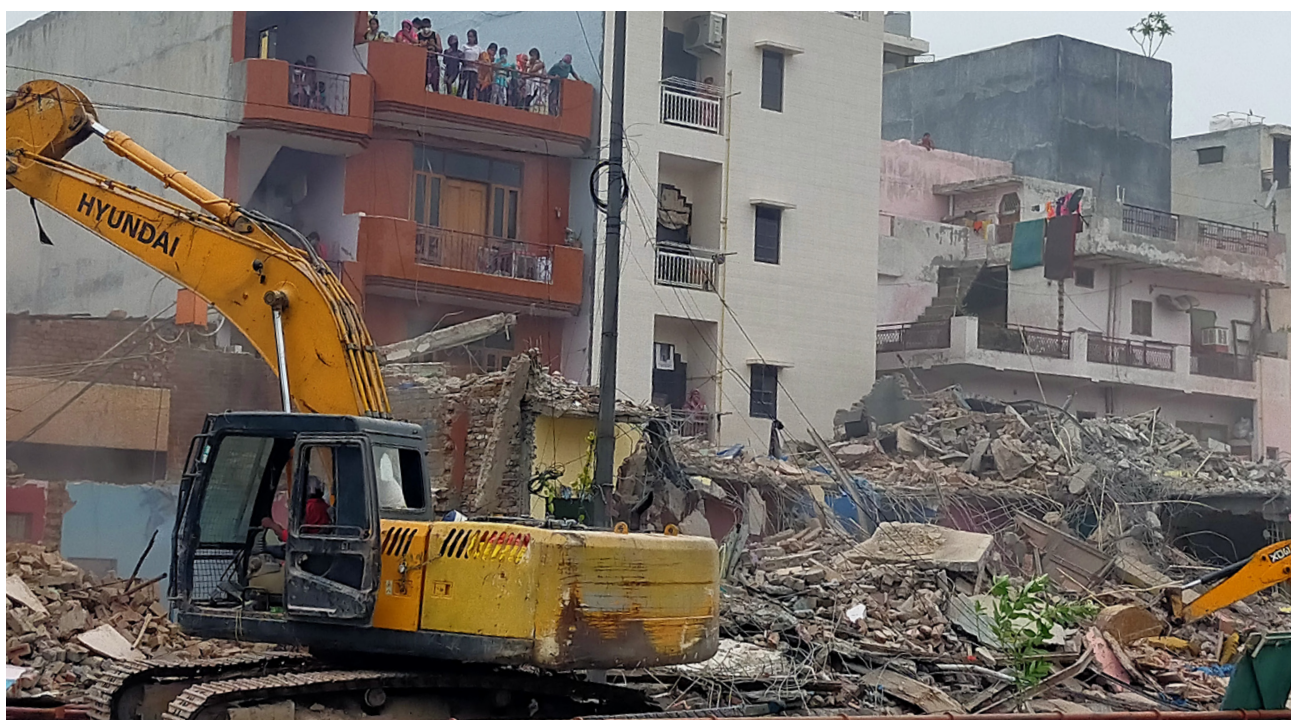
Demolition drive at East Laxmi Market, Delhi
