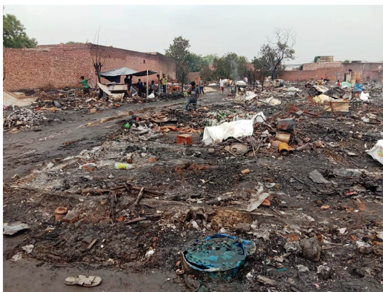
Gutted homes, Shahabad Dairy, Delhi
