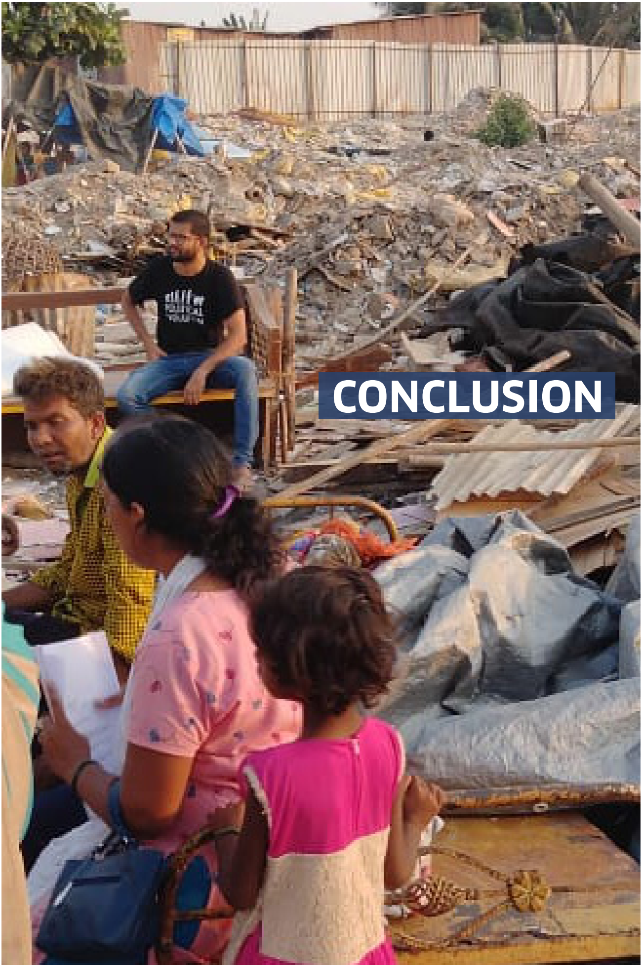
Demolition in Charkop, Mumbai
