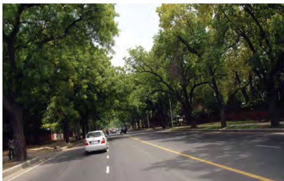
FIGURE 6.7 Trees along road
