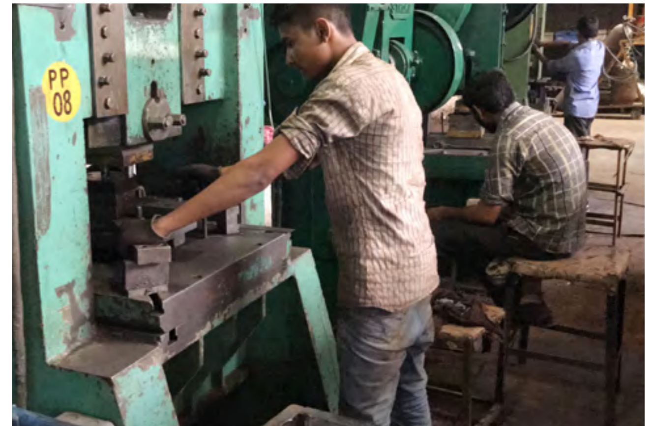
A typical poorly maintained power press, where more than half of such accidents occur.
